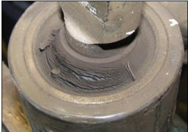
Figure 5-8; Acceptable surface cracks
